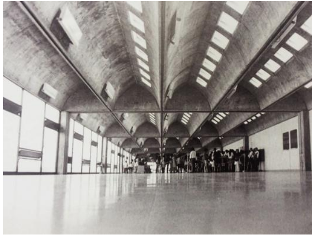
Figura 04 – Hospital Taguatinga – Sheds
